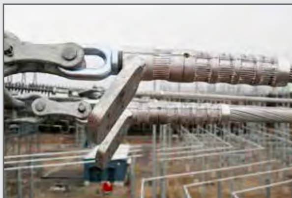
Only 4 Swages required on AAC Single Pad Deadends
