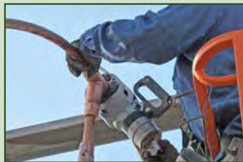
The lightweight Swage Tool connects cables in even the most hard to reach places
